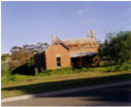
SD 190 - House, Navarre Street (corner Albert Street), ST ARNAUD
