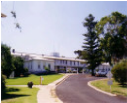
SD 192 - St. Arnaud Hospital, North Western Road, ST ARNAUD
