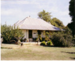
SD 202 - House, 3 Outram Street, ST ARNAUD
