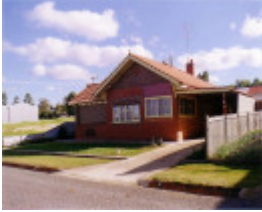
SD 205 - House, 5 Queens Avenue, ST ARNAUD
