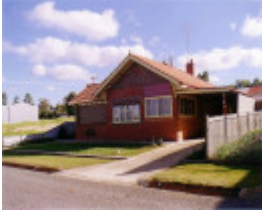
SD 205 - House, 5 Queens Avenue, ST ARNAUD
