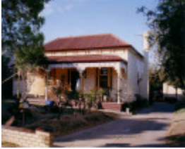
SD 206 - House, 10 Queens Avenue, ST ARNAUD
