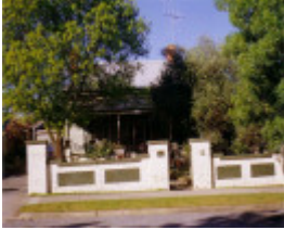
SD 207 - House, 12 Queens Avenue, ST ARNAUD
