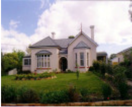
SD 215 - House - 'Symington House', 29 Queens Avenue, ST ARNAUD
