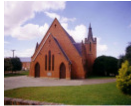
SD 218b - view showing bell tower. Note entry gable is a later addition.
