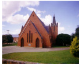
SD 218b - view showing bell tower. Note entry gable is a later addition.
