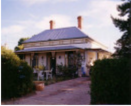
SD 219 - House, 31 Queens Avenue, ST ARNAUD
