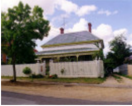
SD 220 - House, 32 Queens Avenue, ST ARNAUD
