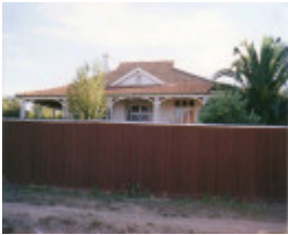
SD 221 - House - 'Waroongah', 35 Queens Avenue, ST ARNAUD
