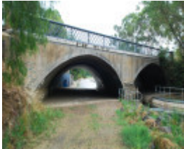
KINGS BRIDGE, OVER BENDIGO CREEK SOHE 2008
