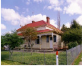
SD 227 - House, 53 Queens Avenue, ST ARNAUD
