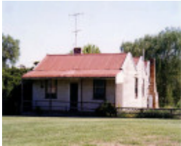
SD 230 - House, 67 Queens Avenue, ST ARNAUD
