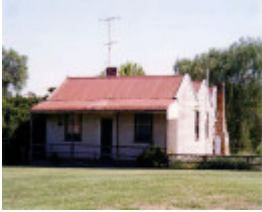
SD 230 - House, 67 Queens Avenue, ST ARNAUD
