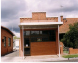
SD 231 - Brick shop, Raglan Street, ST ARNAUD
