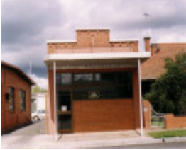
SD 231 - Brick shop, Raglan Street, ST ARNAUD
