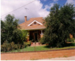
SD 233 - House- 'Lenlethan', 3 Raglan Street, ST ARNAUD
