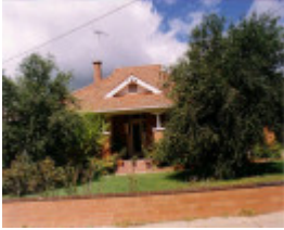
SD 233 - House- 'Lenlethan', 3 Raglan Street, ST ARNAUD
