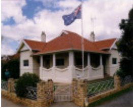
SD 234 - Preece House, 5 Raglan Street, ST ARNAUD
