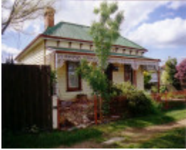
SD 236 - House, 10 Raglan Street, ST ARNAUD
