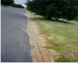
SD 248 - Brick Street Gutters, Silvermines Road, ST ARNAUD
