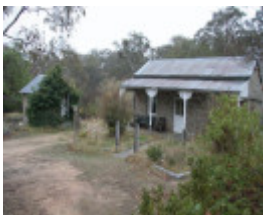
PROV H2127 Granite Cottage
