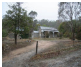
PROV H2127 Granite Cottage
