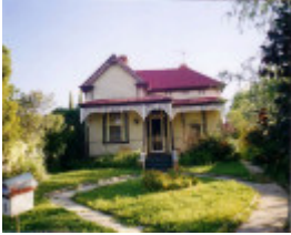
SD 257 - House, 9 Victoria Street, ST ARNAUD
