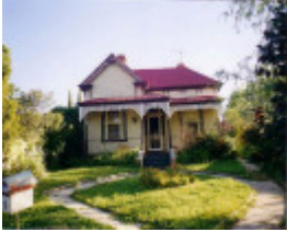
SD 257 - House, 9 Victoria Street, ST ARNAUD
