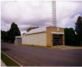
SD 258 - St. Arnaud Fire Station, Walker Street (corner Dundas Street), ST ARNAUD
