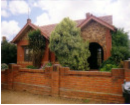
SD 260 - House, 4 Walker Street, ST ARNAUD
