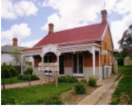
SD 261 - House, 6 Walker Street, ST ARNAUD
