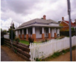
SD 262 - House,8 Walker Street, ST ARNAUD
