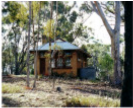
SD 264 - Former St. Arnaud East School No 2389, Wedderburn Road, ST ARNAUD
