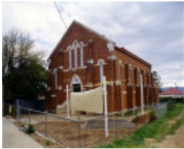
SL 002a - Stawell Scout Hall (former St. Mark's Presbyterian Church), 20 Alfred Street, STAWELL
