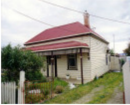
SL 005 - House, 24 Allen Crescent, STAWELL
