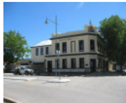
Former Bank of NSW
