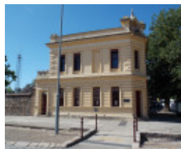
Bank of NSW south side
