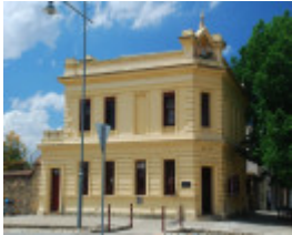
BEECHWORTH WINE CENTRE SOHE 2008
