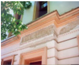
former bank of nsw beechworth facade detail 1995
