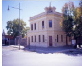
h00349 1 former westpac now bank of melbourne ford street beechworth corner facade she project 2003
