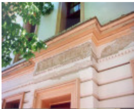
former bank of nsw beechworth facade detail 1995
