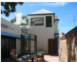
Former Bank of NSW 18 Nov 2014 (25) rear addition
