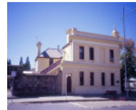
h00349 former westpac now bank of melbourne ford street beechworth camp st facade she project 2003
