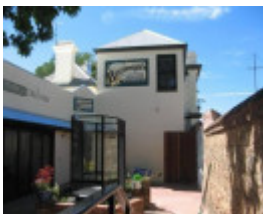
Former Bank of NSW 18 Nov 2014 (25) rear addition
