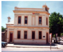
former bank of nsw beechworth front view 1995
