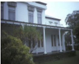
Ulimaroa St Kilda Road St Kilda Verndah View May 1986
