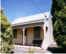
SL 020 - House, 8 Bennett Street , STAWELL
