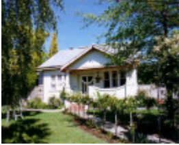
SL 021 - House, 10 Bennett Street, STAWELL
