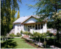
SL 021 - House, 10 Bennett Street, STAWELL
