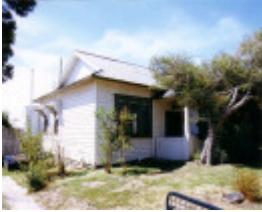
SL 037 - House, 7 Childe Street, STAWELL
