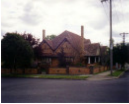
SL 038 - House, 15 Childe Street, STAWELL
