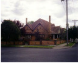
SL 038 - House, 15 Childe Street, STAWELL
