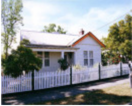
SL 040 - House, 19 Childe Street, STAWELL
