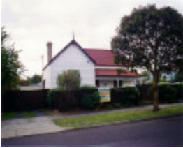
SL 041 - House, 21 Childe Street, STAWELL
