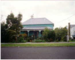
SL 042 - House, 27 Childe Street, STAWELL
