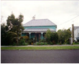
SL 042 - House, 27 Childe Street, STAWELL
