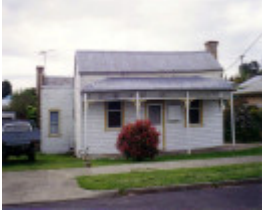
SL 043 - House, 29 Childe Street, STAWELL
