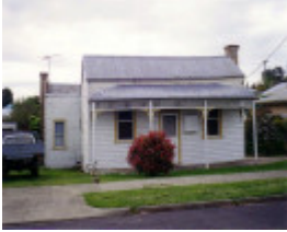
SL 043 - House, 29 Childe Street, STAWELL
