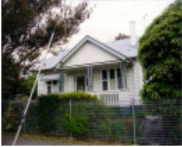
SL 044 - House, 30 Childe Street, STAWELL
