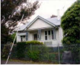
SL 044 - House, 30 Childe Street, STAWELL
