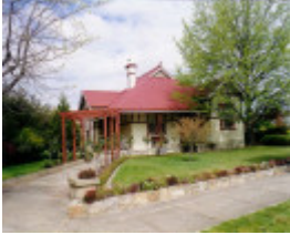
SL 048 - House, 7 Clemes Street, STAWELL
