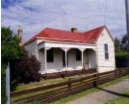
SL 049 - House, 9 Clemes Street, STAWELL
