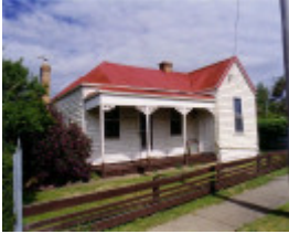
SL 049 - House, 9 Clemes Street, STAWELL
