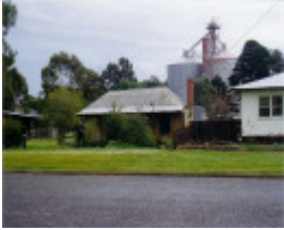
SL 070 - House, 13 Curtis Street, STAWELL
