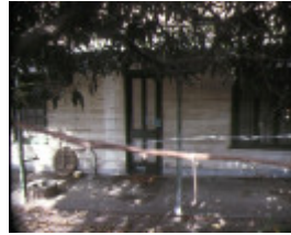
1 residence waterloo crescent st kilda front view
