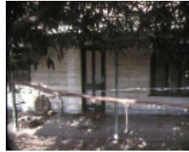
1 residence waterloo crescent st kilda front view
