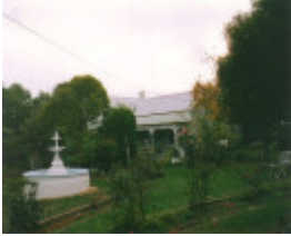
SL 077 - 'Alvie', House, 39 Darlington Road, STAWELL
