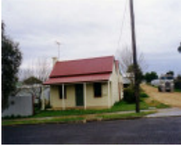
SL 088 - House, 8 Doyle Street, STAWELL
