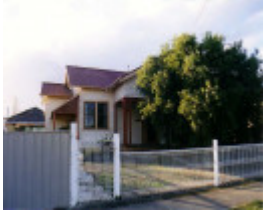
SL 090 - House, 10 Florence Street, STAWELL
