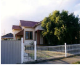
SL 090 - House, 10 Florence Street, STAWELL
