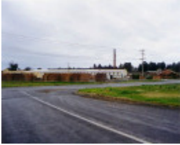
SL 100 - Brickworks, Griffith Street, STAWELL
