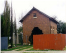
SL 101 - Former Police Stables, Griffith Street, STAWELL
