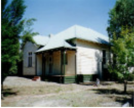
SL 118 - House, 3 Johnson Street, STAWELL
