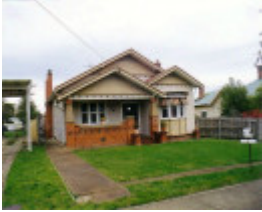
SL 120 - House, 7 Johnson Street, STAWELL
